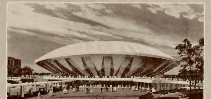
ASSEMBLY HALL — UNDER CONSTRUCTION
