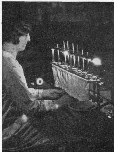
—Cut courtesy Westinghouse. DRILLING DIAMOND DIES
