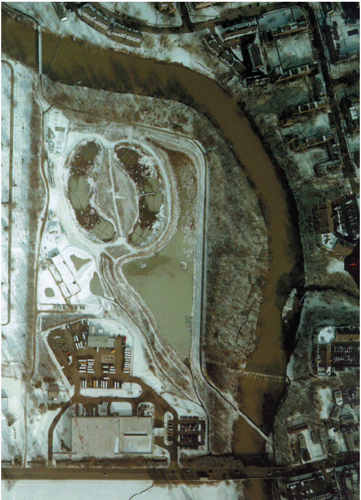
Figure 3. Aerial photo of entire site on January 8, 2003, about 31 months after levees were cut.
