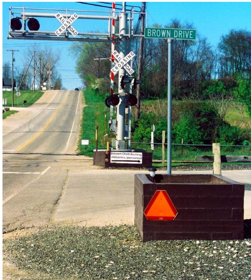
Figure 5: A Slow-Moving Vehicle Emblem Incorrectly Used (Ohio)
