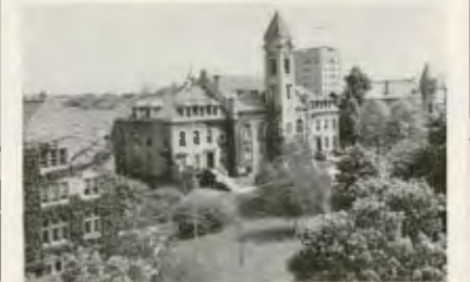
LIBRARY, STUDENT BUILDING
