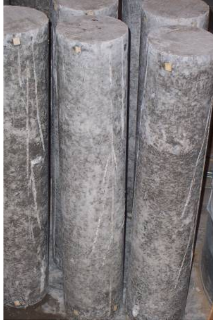
Figure 3.1 – Base Columns Before Retrofitting (Miller 2006).
