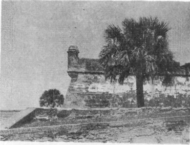
FIGURE 4. Coquina rock was used as the primary building material for Castillo de San Marcos, St. Augustine, Florida.
