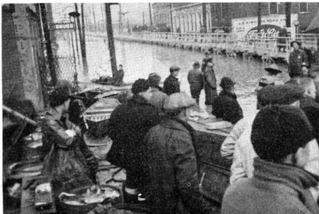
A FLOODED STREET SHOWING TEMPORARY BRIDGE
