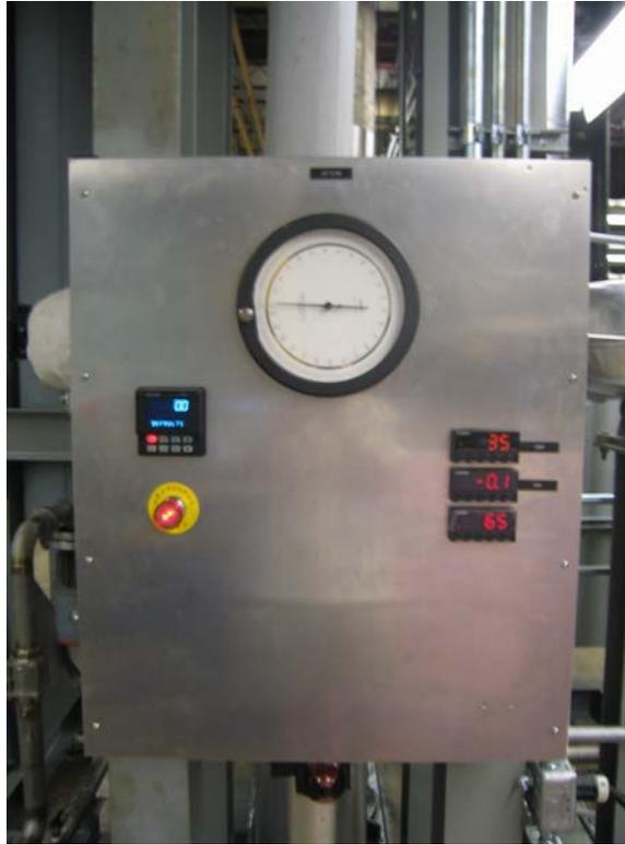
**Figure 3.3 – The control panel used to control the GDTL jet facility. The control system allows for automatic control of the jet stagnation pressure in order to provide a constant Mach # flow.**
