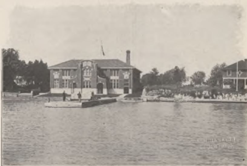
FISH HATCHERY, FRONT VIEW
