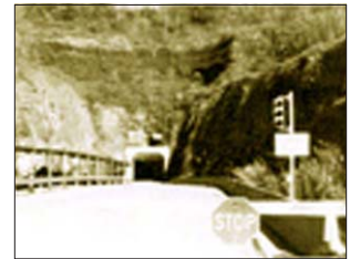
Underground storage entrance
