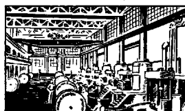
MAKING THE CABLE
